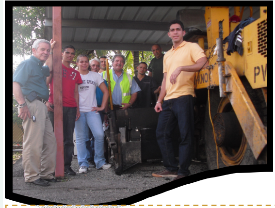
Installation of Ramp Champ (from left to right): Ramón Caunabo (Betterroads), Reinaldo Silvestry (M.Eng. UPRM), Leilany Benejam (BS Purdue), Eric Rivera (BS PUPR), Benjamín Colucci (PR-LTAP), Daniel (Betterroads) and Freddie Salado (M.Eng., UPRM).
