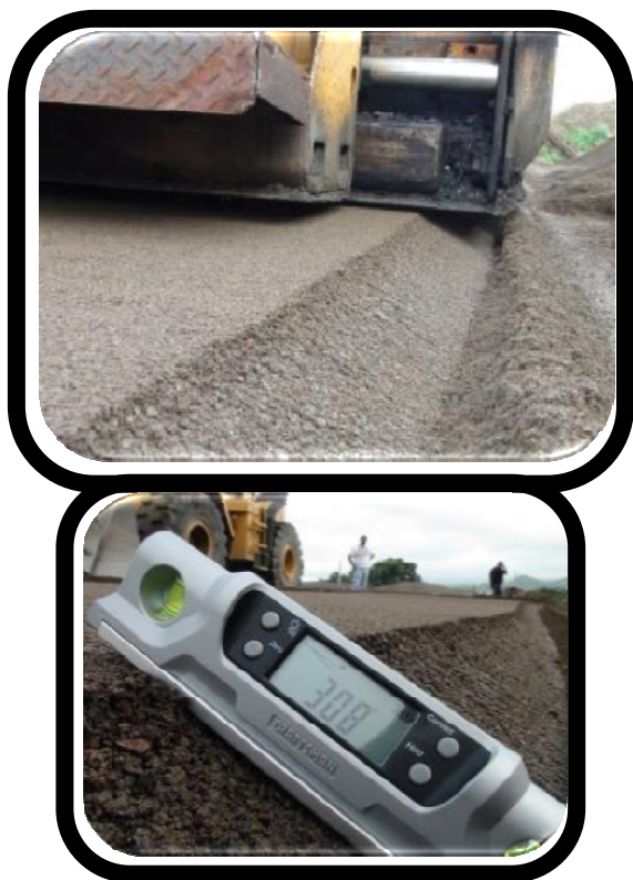
Pictures from the Test Site of the Safety Edge on the Robles Asphalt Plan.
